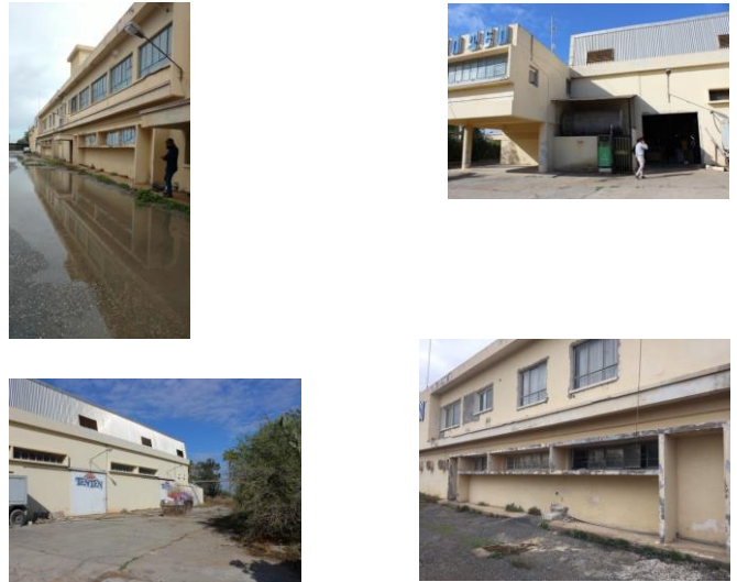
Fig.3. current situation of building taken by: Hesam Mosharraf
